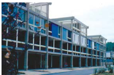
Hickory Cluster Town homes, completed model, front exterior, May 1965
