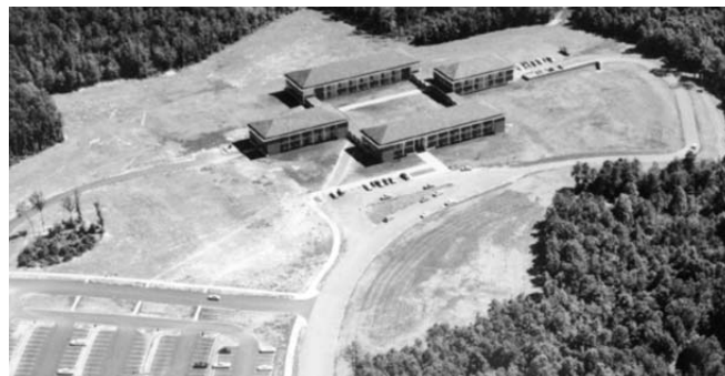
Fairfax Campus circa 1964, showing the original four buildings: North [now Finley], South [now Krug], East, and West (photograph source: George Mason University Archives)
